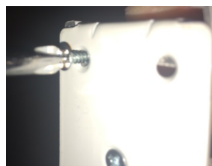
Slide bracket wings all the way into the headrail and attach with provided screws
