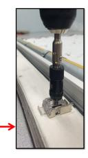
17. Snap the head rail into the mounting brackets.
