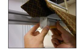
24. Test the shade. Pull the shade all the way down to the lower position. Now tug and release ring and watch the shade go back up to the stop position that you just set.
