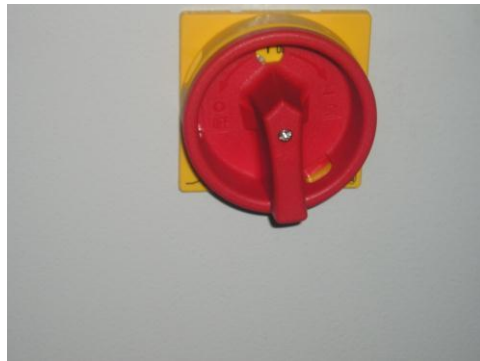
Picture-2 Power Isolator switch
