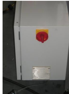
Picture –3 Power Isolator
